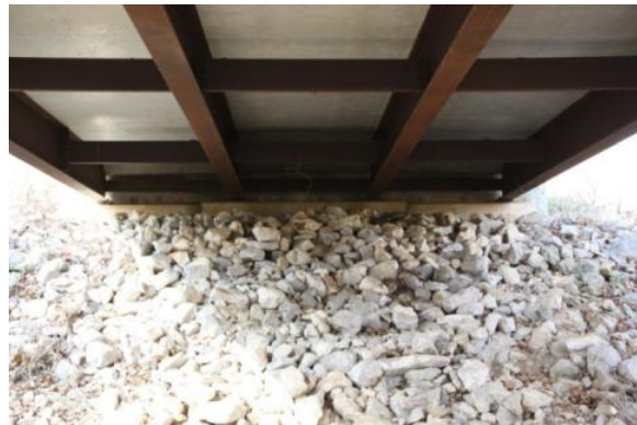
Figure 7.2. Photographs showing typical pier (left) and typical abutment (right). (Photos by EVF, Fayetteville, 10/18/13)
