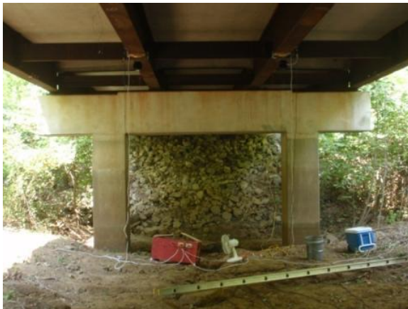
Figure 7.2. Photographs showing typical pier (left) and typical abutment (right). (Photos by EVF, Fayetteville, 10/18/13)
